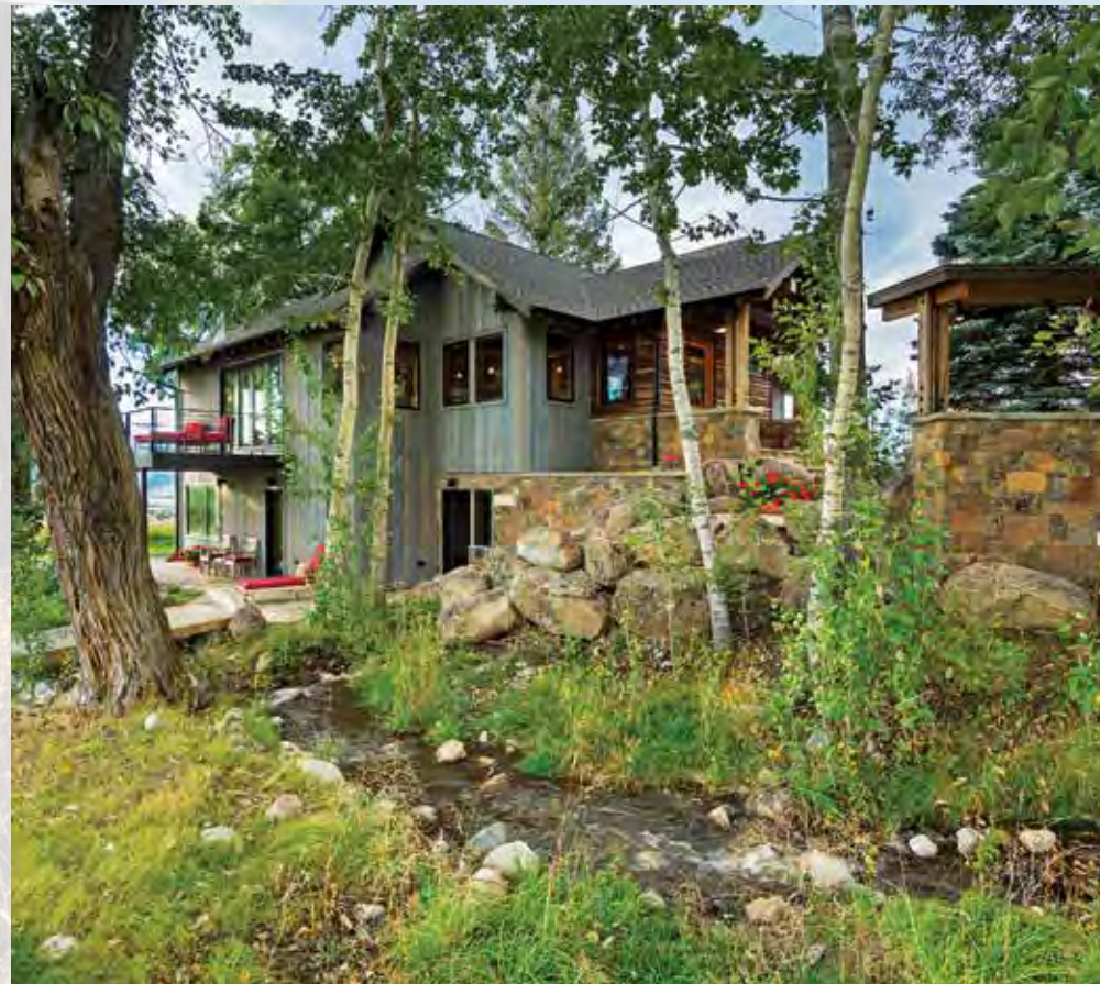
ABOVE: The homeowners wanted the outdoors to feel like a part of their home environment. A quick trip outside to cook dinner on the grill helps achieve this effect. RIGHT: The design team worked together to remove the old farmhouse and modernize the foundation, which had previously flooded and was sheltering "a pretty hardy mouse population," according to Rudolph. The home's footprint remained essentially the same even while the flow and functionality were substantially improved.
